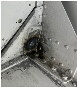
Steel side welded
